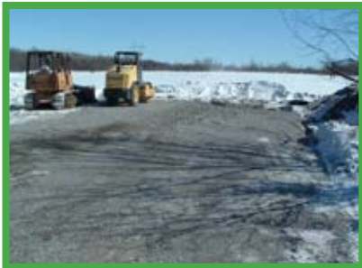
Completed road to the Ryan Substation, facing east of Ryan Rd.
