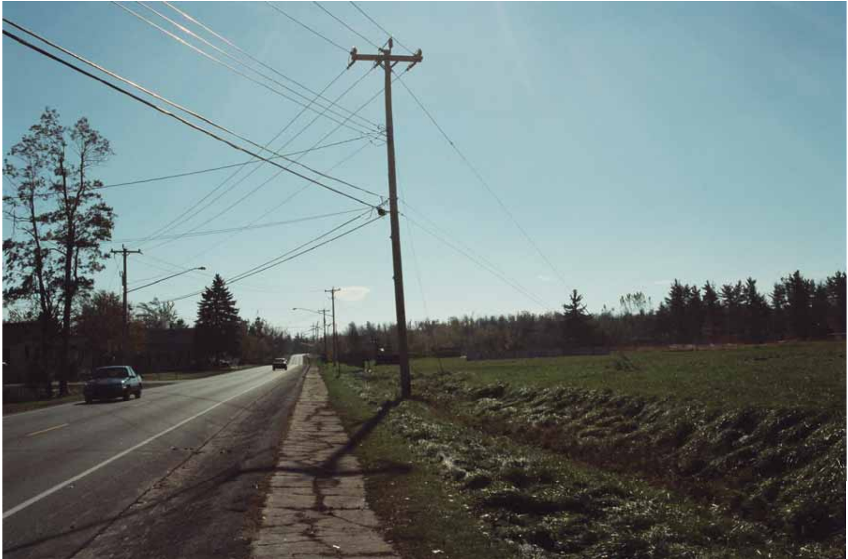
Viewpoint G: Devil's Den Road, in Front of Feinburg Park, Altona, facing south
