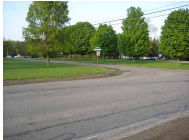
3b. Richardson Rd at Taylor Collo Rd Looking SW
