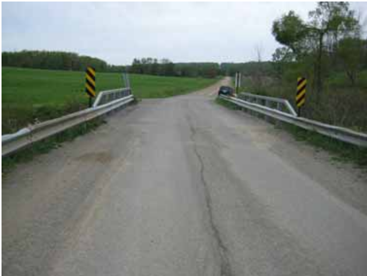
1 c. Wentworth Rd Bridge Looking North
