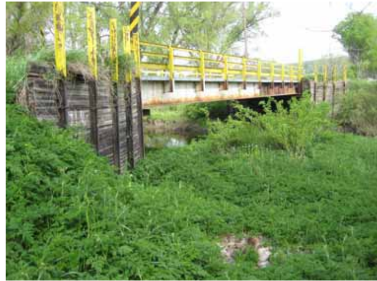
1 b. Cemetery Rd Bridge Looking NW
