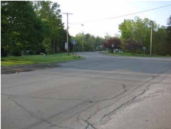
3c. Taylor Collo Rd at Route 3 S Looking South
