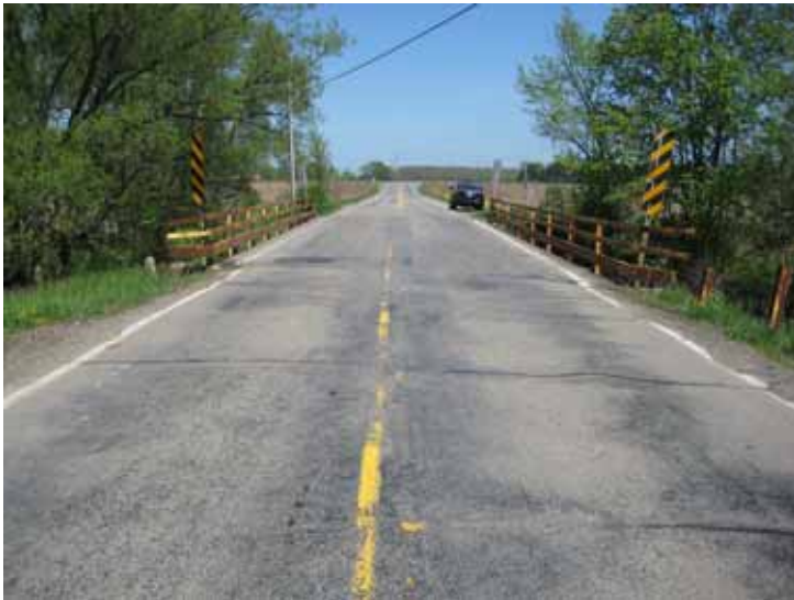
14c. Balcom Cross Rd Bridge Looking North
