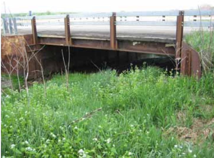
12c. Buttermilk Rd – Small Bridge Looking SW
