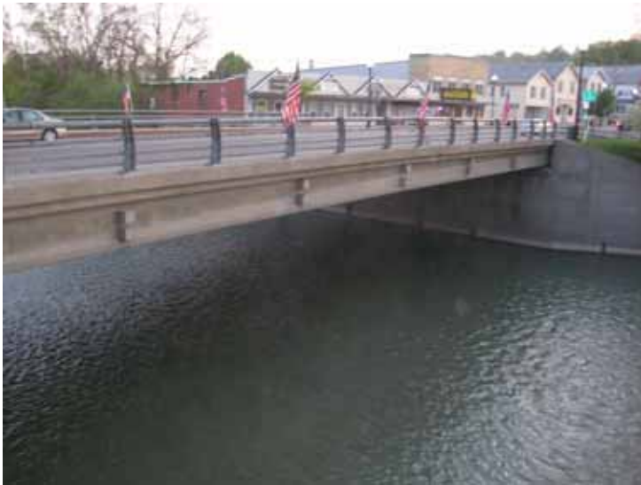
a. Otonda Bridge Looking SW
