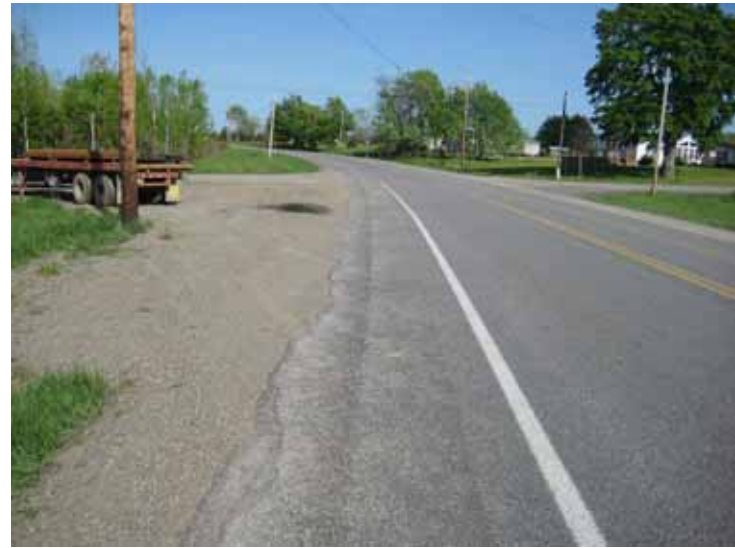
10b. Route 39E at Empire Rd – NW Access
