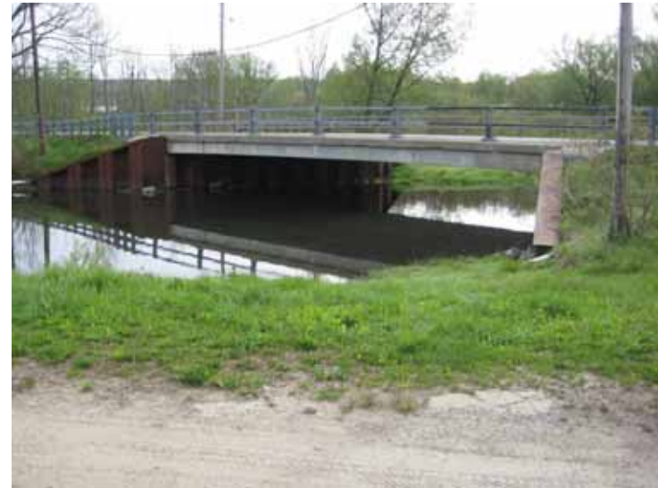
12b. Buttermilk Rd – Big Bridge Looking SW
