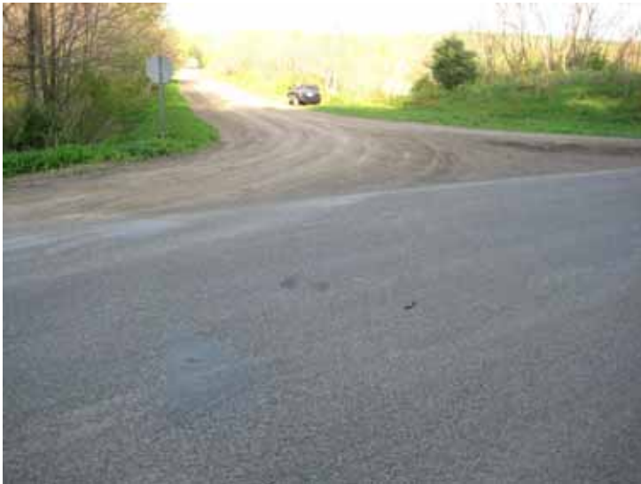
11c. East Lake Rd at Mye Rd Looking East
