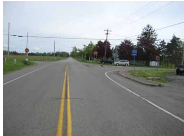
d. Route 39W at Stafford Rd Looking South
