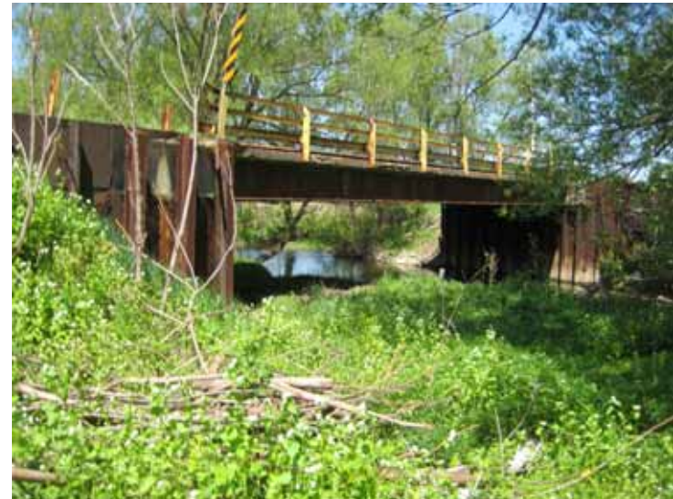
14d. Balcom Cross Rd Bridge Looking NW
