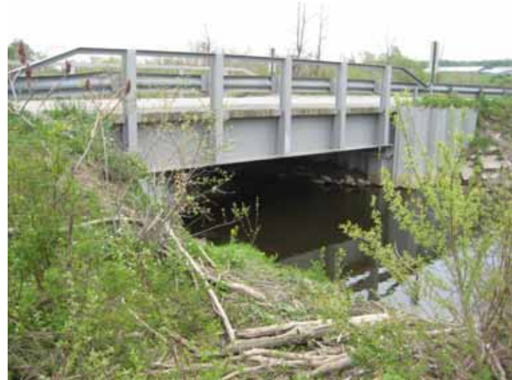
1 d. Wentworth Rd Bridge Looking SE
