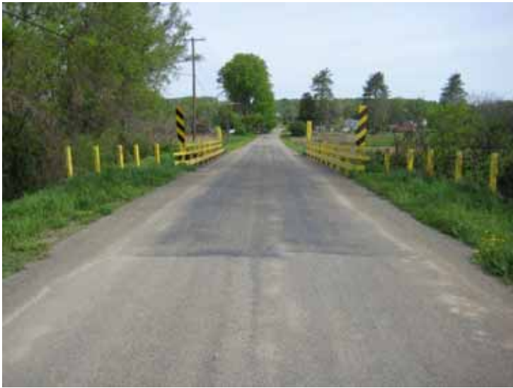
1 a. Cemetery Rd Bridge Looking North
