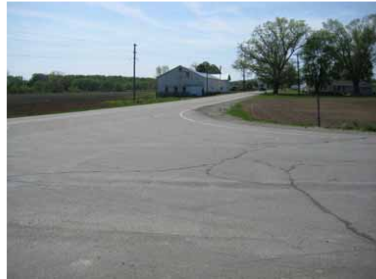
13b. Butterilk Rd at Hooker Rd Looking SW
