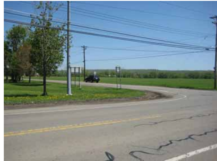
14b. SR83 at Balcom Cross Rd Looking NE
