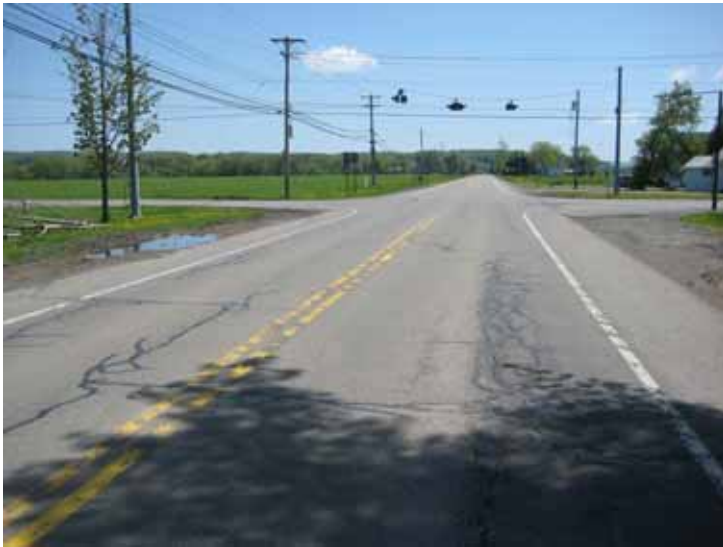
14a. SR 38S at Balcom Cross Rd (CR87) Looking East
