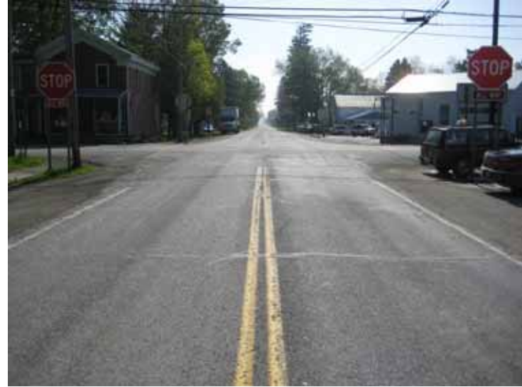
6d. Route 62N, Ellington Center - South Access
