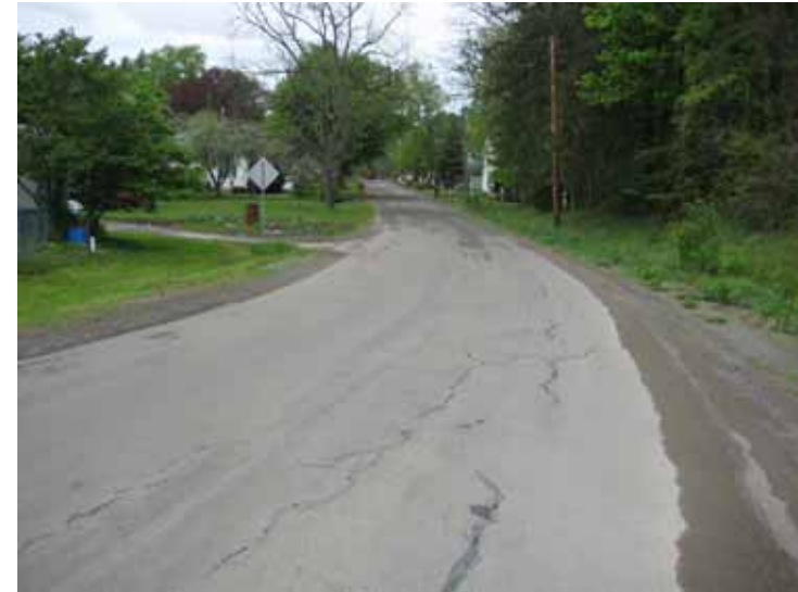
1d. Collins Rd By-Pass Looking West
