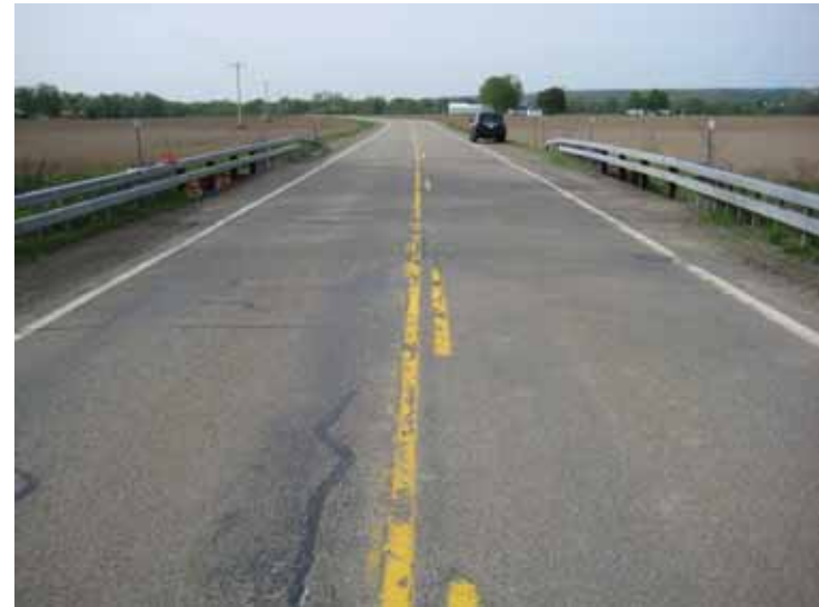
12d. Buttermilk Rd – Small Bridge Looking South
