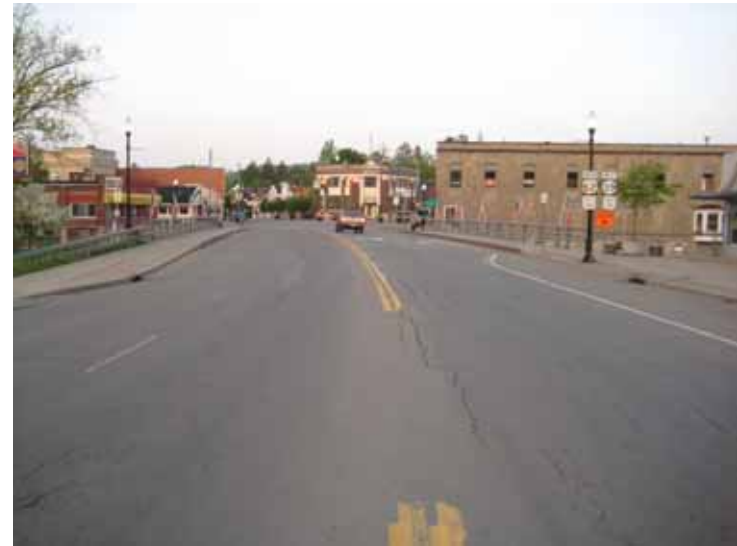
4d. Gowanda Bridge over Cattaraugus Creek
